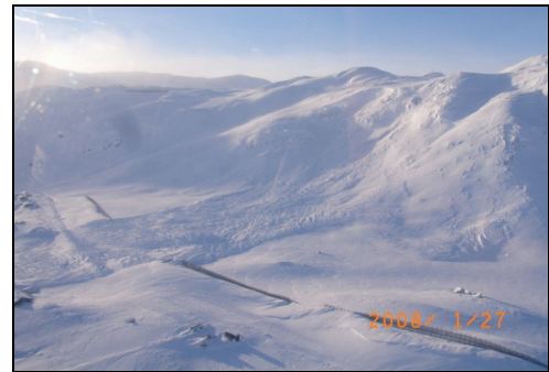
Figure 4: Avalanche event in January 2008 in the Tyin area, Central Norway. Avalanches were naturally released in the period from 24.01.2008 to 26.01.2008. Road closure lasted for approx. 3 days. Upper picture: manually recorded avalanche events on and along Fv53 (Map source: NPRA). Lower picture: oblique photograph of a snow avalanche crossing the road. The avalanche had descended from right to left, first crossing the snow drift fence, then the road and finally destroying one building. (Photo by Svein Helge Frækaland, NPRA Region west, 27.01.2008).
